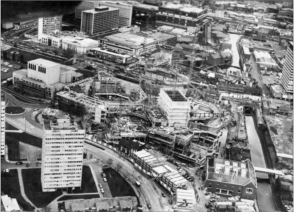
THE INTERNATIONAL CONVENTION CENTRE AND SYMPHONY HALL UNDER CONSTRUCTION
